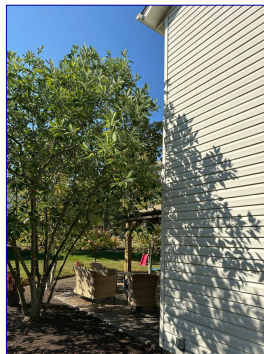
There is vegetation in contact with the house. Recommend trimming trees/vegetation, so it is doesn't come into contact with the home.
