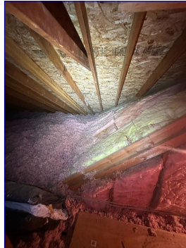
Attic in Home.
