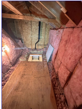
Havoc access from master closet
