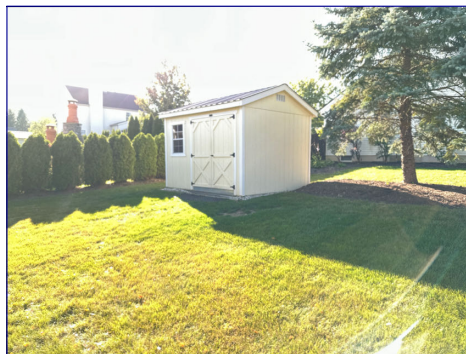
Outbuildings are not part of the home inspection.
