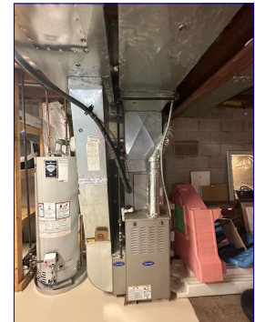
The furnace area
