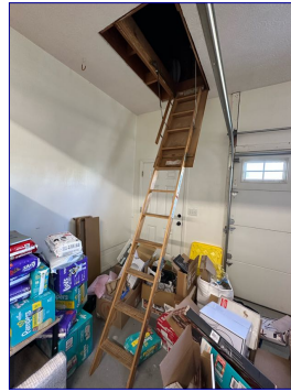
Attic pool downstairs to garage attic.
